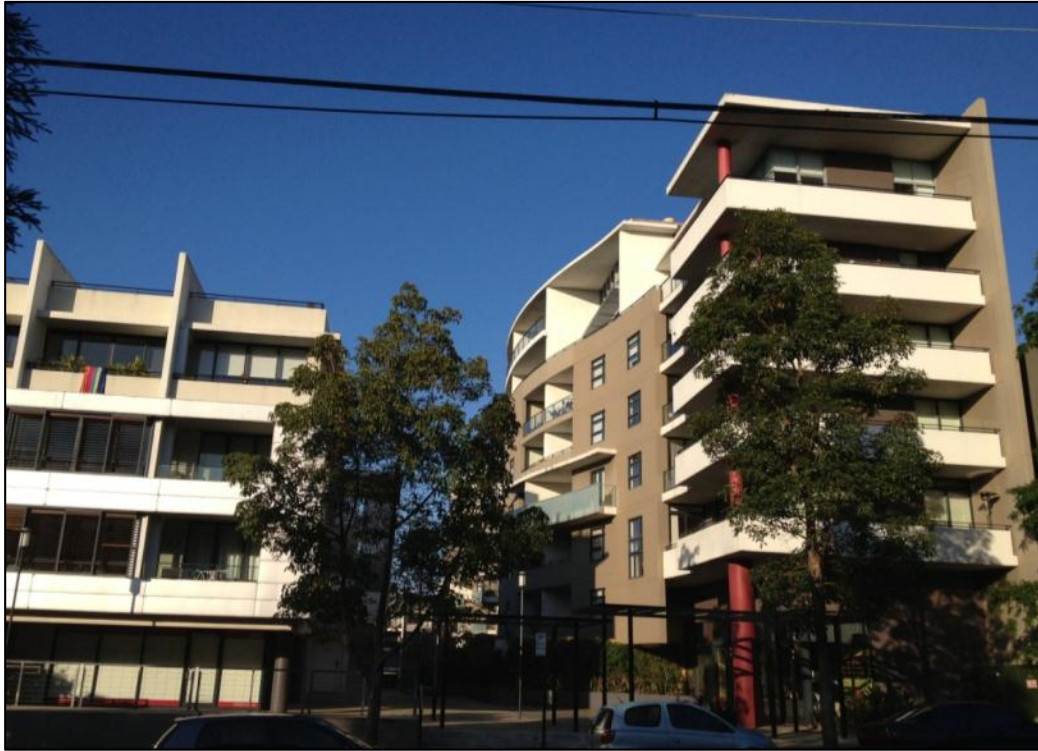
Figure 9: The 4-7 storey mixed use development (known as 1-5 and 7-11 Hunter Street) located to the east of the site
